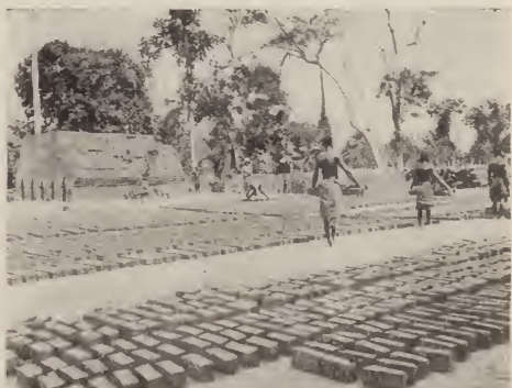
The brickyard at Luebo, in charge of Mr. Hillhouse. Making bricks for the hospital and training school.
